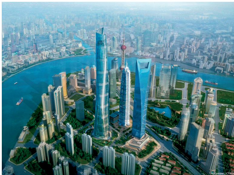
Rys. 8. Shanghai Tower, http://skyscrapercenter.com/building/shanghai-tower/56
